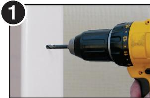
1 Drill 5/16" hole through your post. Counterbore with 1/2" drill on inside face if embedding Quick-Connect® body.
