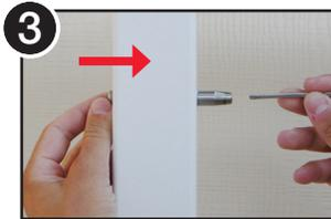
3 Thread bolt through post and 1/2" into Quick-Connect® fitting. Insert cable all the way into Quick-Connect® fitting, until it stops.
