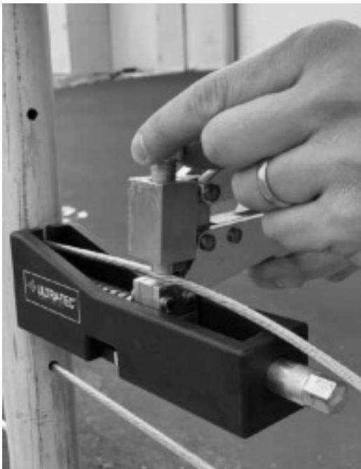
3. Using an impact driver with ½" socket, tighten the cable to the desired tension — for best results, lightly apply lubricant to the threads. The indications in the load window are for reference only; a tension gauge is required for accuracy.
