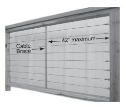
As indicated above, this support can be provided with intermediate posts or a lighter material acting as a cable brace. As with an intermediate post, a cable brace also runs between the top rail and the lower mounting surface, but its purpose is only to support the cable. It is not intended to be an element providing structural support to the railing.
