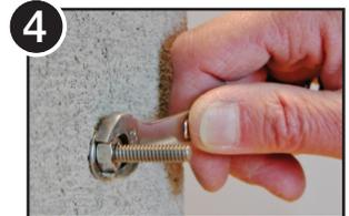
4 Use 7/16" wrench to tighten anchor nut until anchor is properly seated and locked.
