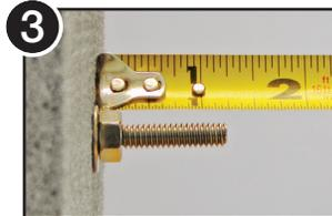
3 Tap until approximately 1-1/4" of the threaded shaft protrudes from the wall.
