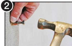
2 Carefully tap the Expansion Anchor (with washer & anchor nut).
