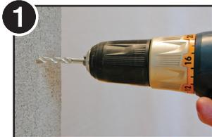
1 Drill 1/4" hole with masonry bit to 1-1/4" (minimum) depth. Blow debris out of hole.
