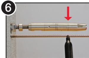
6 Stretch cable tight across fitting and mark at Cut Gauge Line. Cut cable at mark.
