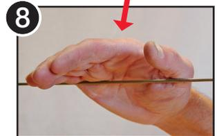
8 Hand tighten the Quick-Connect® as far as possible, then swiftly hit the cable line with your palm several times to ensure that jaws are securely seated.
