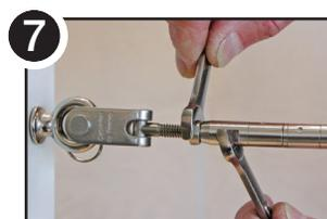
7 Tighten the lock-nut against the Quick-Connect® to prevent the fitting from loosening
