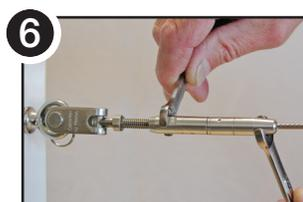
6 Use 3/8" wrenches to tighten the Quick-Connect® to desired final tension.
