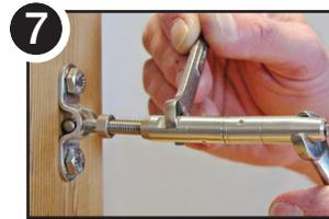
7 Use 3/8" wrenches to tighten the Quick-Connect® to desired final tension.
