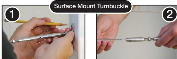
1 Measure, mark and drill pilot holes. Bolt/screw Surface Mount Turnbuckle to wall.
