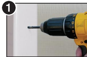
1 Drill 5/16" hole through your post. Counterbore with 1/2" drill on inside face if embedding Quick-Connect® body.
