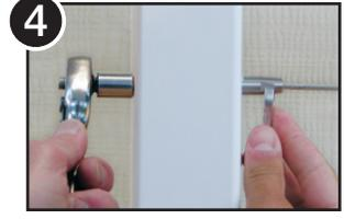
4 Tighten the nut to tension the line. Use wrench to prevent the Quick-Connect® from rotating during tensioning.
