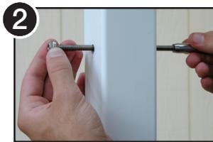
2 Attach washer and nut, leaving room for final tensioning of fitting & cable.
